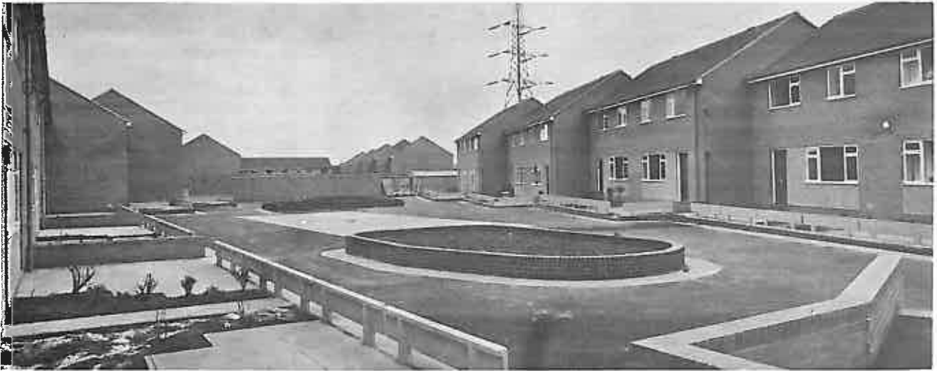
HOUSES AND GARAGES ON THE PERCY MAIN REDEVELOPMENT SITE BUILT FOR TYNEMOUTH C.B.C.
