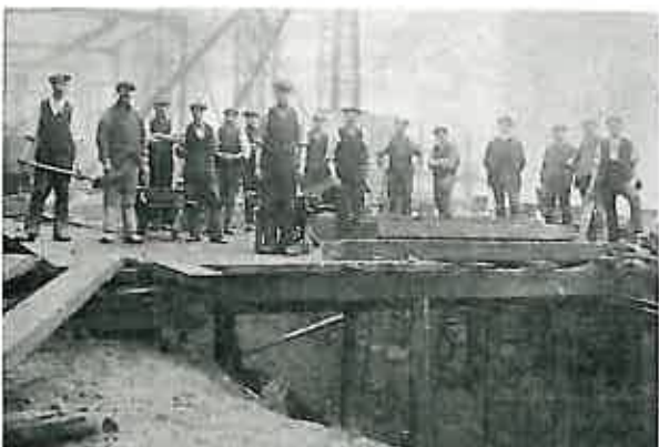
DOXFORDS RETAINING WALL WITH PERSONNEL 1912
