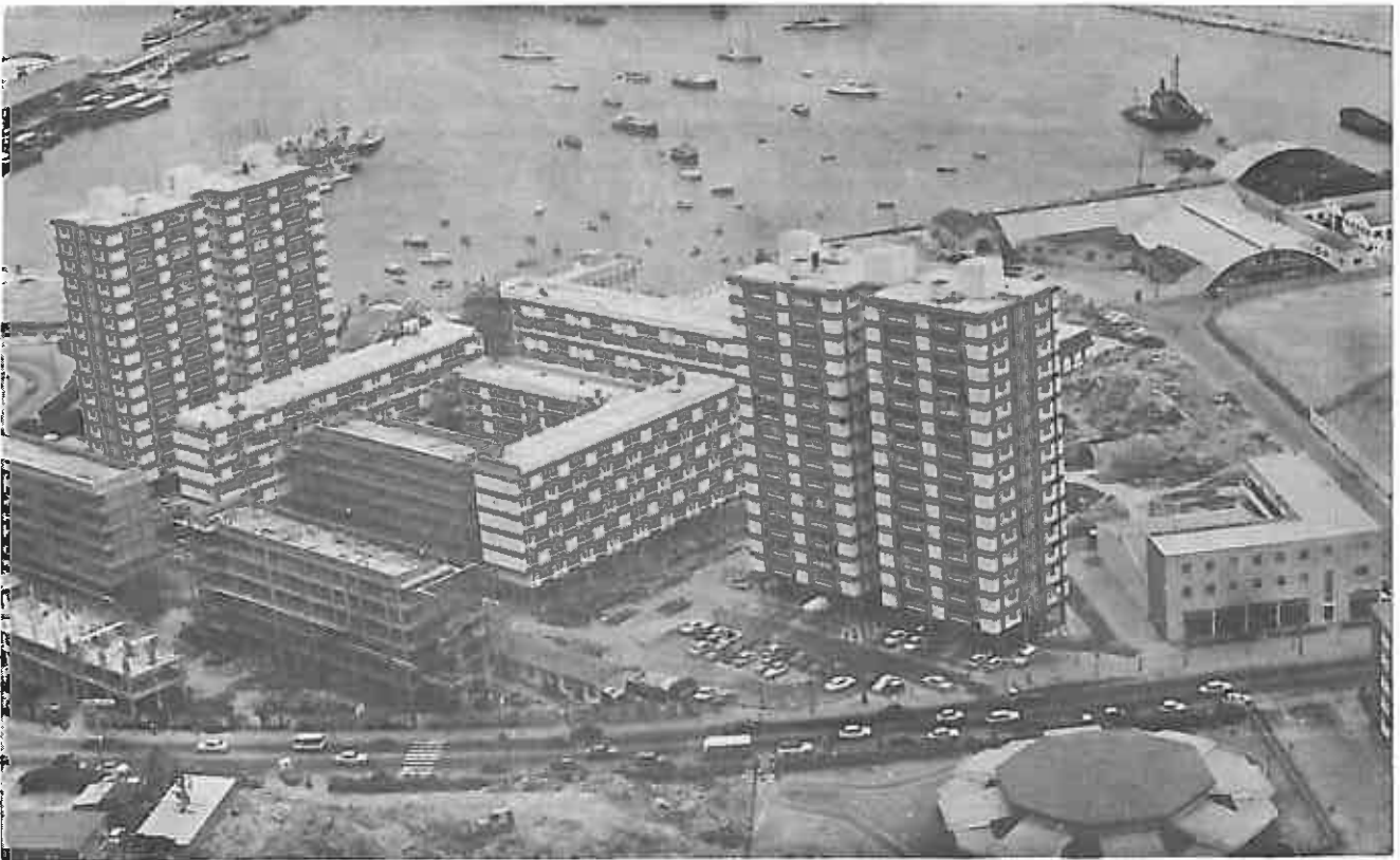
GENERAL VIEW FROM CAROLINES BATTERY
