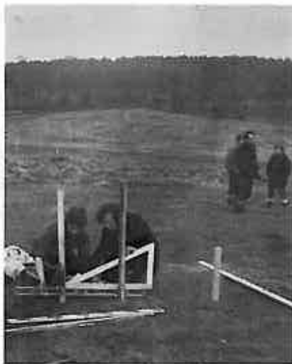
ESTABLISHING TOE OF BATTER
