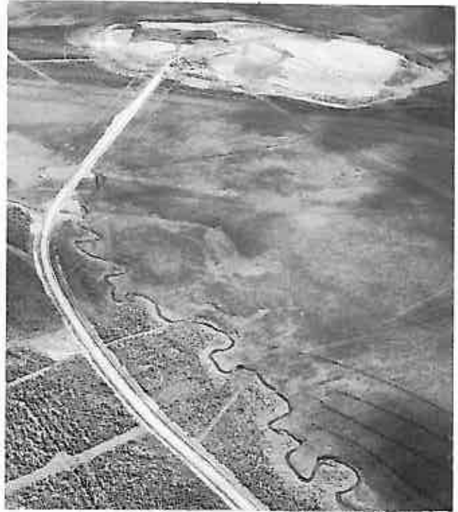
Above:— An aerial view of Berry Hill with part of the R.51 Access Road approach across the deep peat bog which surrounds Berry Hill like sea around an island. The hill has been reduced to form a plateau approx. ½ mile across. A 2m thick layer of peat and soft clay unsuitable had to be cleared off the whole area as an integrated operation with the cut and fill of the good clay underneath. A team of 3 No. 54RB draglines, 8 No. D.8 and scrapers, loading shovels and Volvo dumptrucks plus probably one of biggest ever concentrations of "bog-track" dozers have handled some 300,000 cu.yds. of unsuitable (disposed of on to the peat bog) and 440,000 cu.yds. of cut to fill in 15 weeks. It is hoped that by the end of November, a total of ½m cu.yds. of unsuitable and ½m cu.yds. of suitable will have been handled on the contract as a whole.
